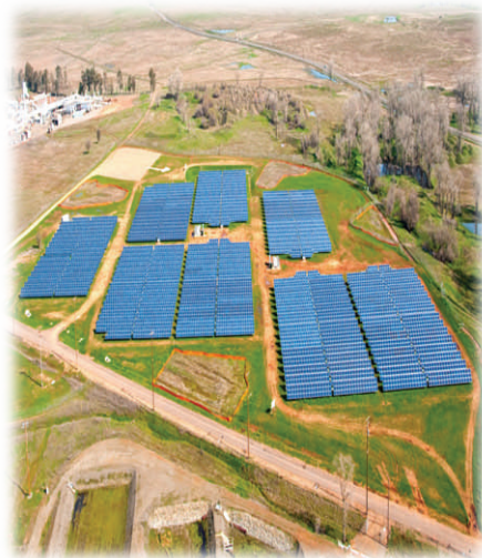
Solar Power Inc. solar farm.
