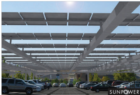
Ventura County parking lot solar system.
