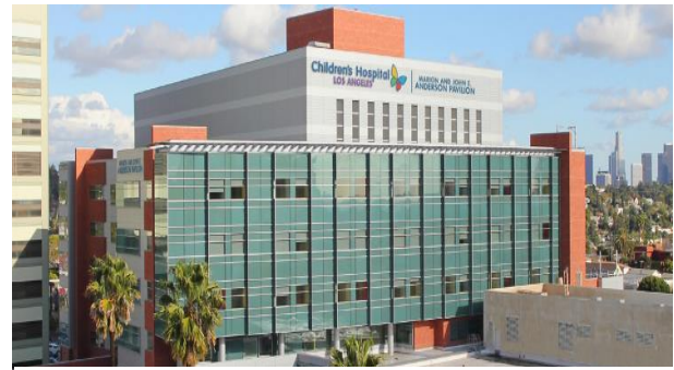
Children’s Hospital Los Angeles – Anderson Pavilion Photo courtesy of Children’s Hospital Los Angeles
