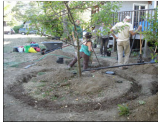
Greywater System Installation
