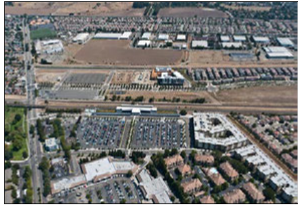
Union City Station District 2011
