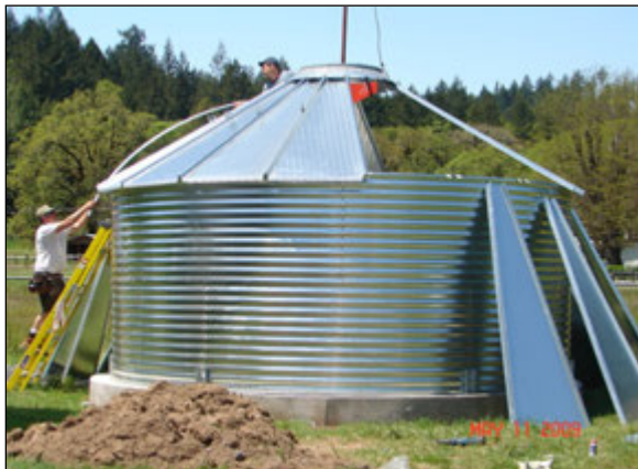
Rainwater Tank Construction
