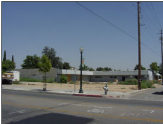
Pre-DEMOLITION of site on Baker Street
