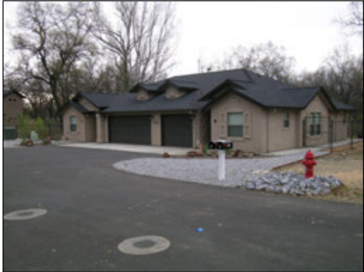
View of newly built duplex
