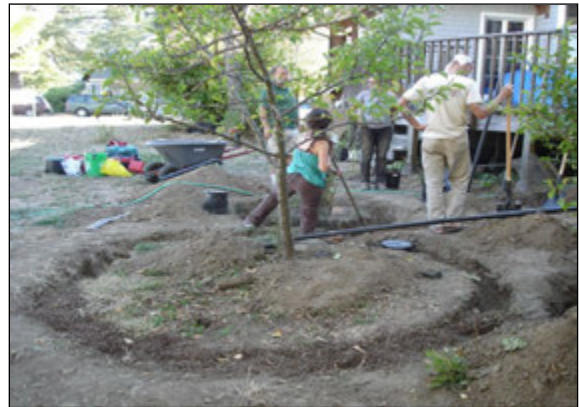
Greywater System Installation
