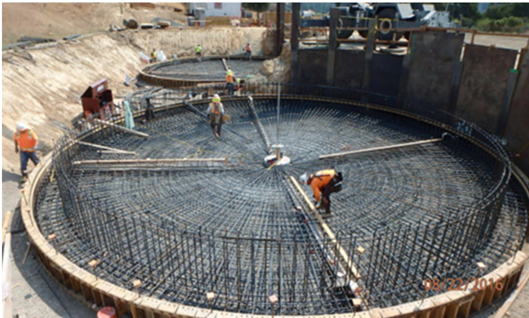
San Jose Water Company project under construction. (Photo Credit: CPCFA)
